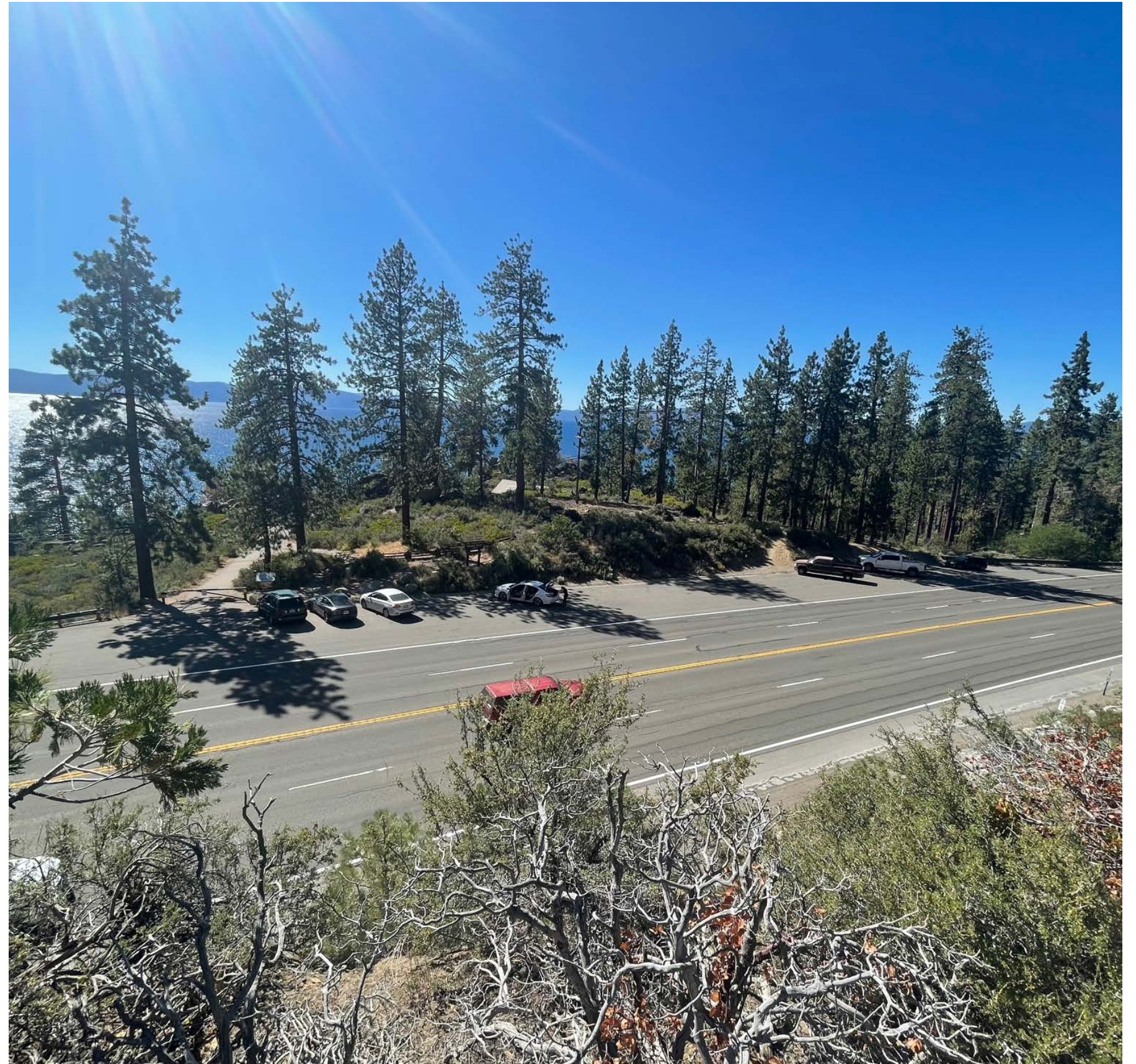
Existing Conditions at Logan Shoals Vista Point
