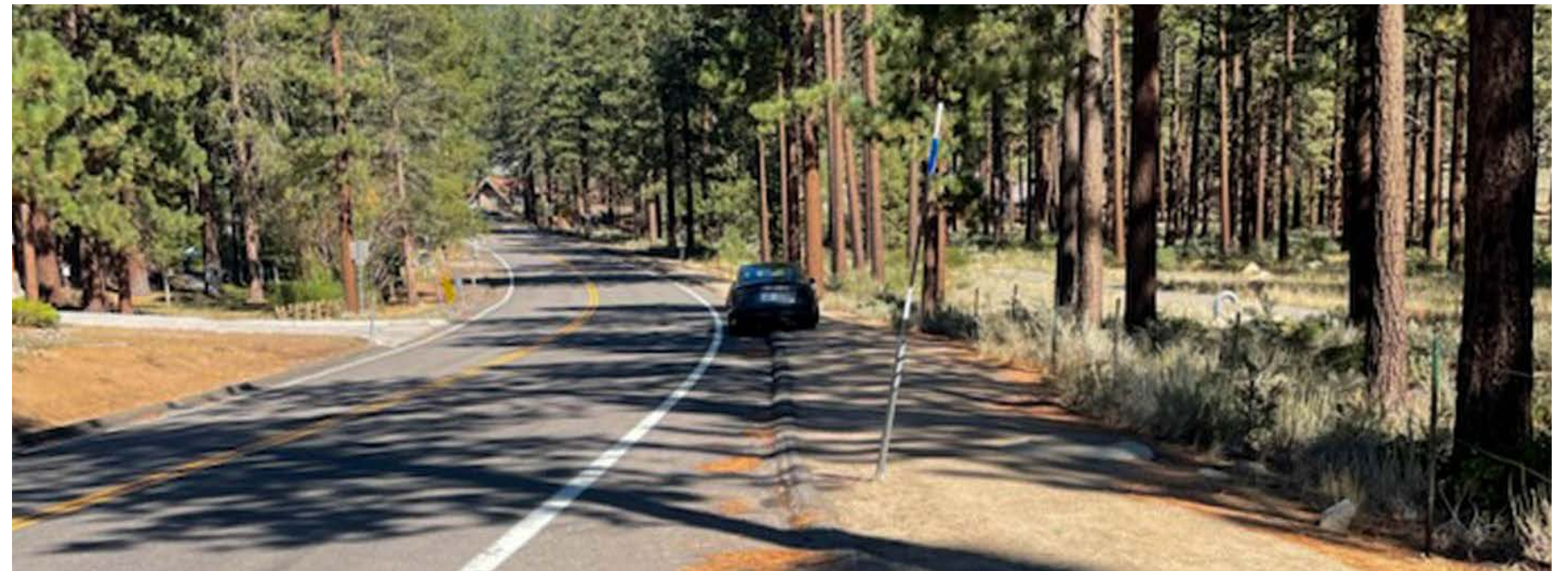
Existing image of parallel parking area
