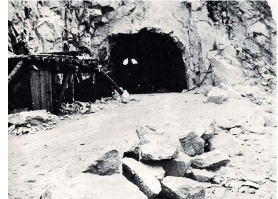
1930s construction of the tunnel at Cave Rock. Source: parks.nv.gov
